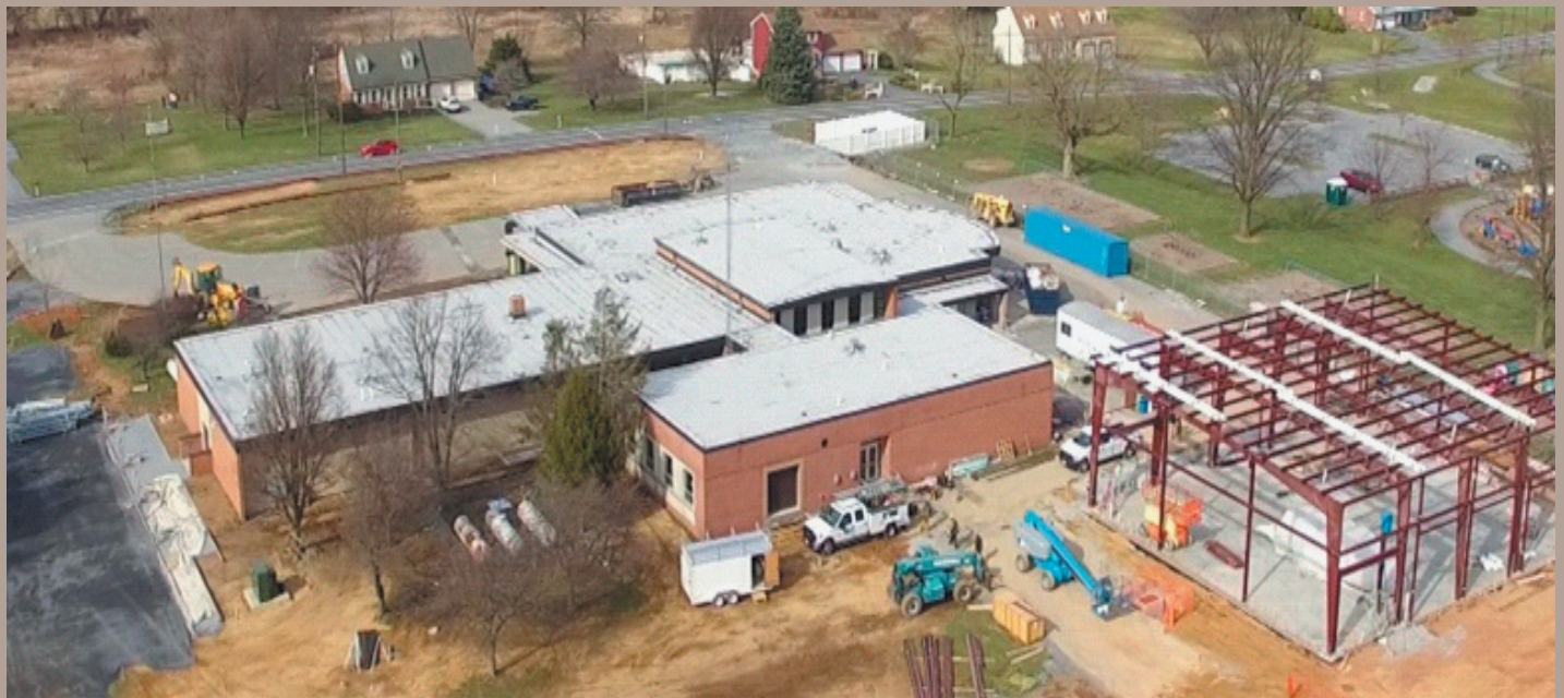
Aerial view of the Mount Joy Twp Municipal Complex under construction
