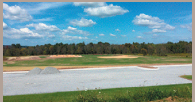
Old Trolley Line Park under construction
