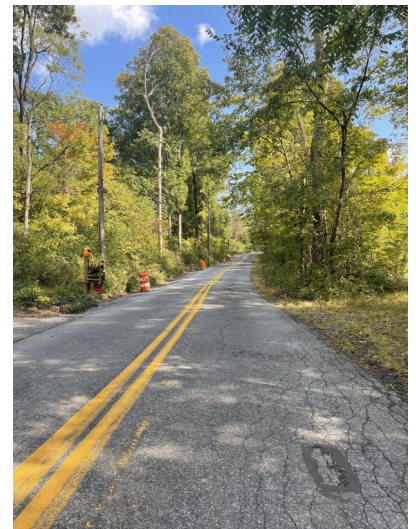
Third and final segment of Trail Road North improvements underway
