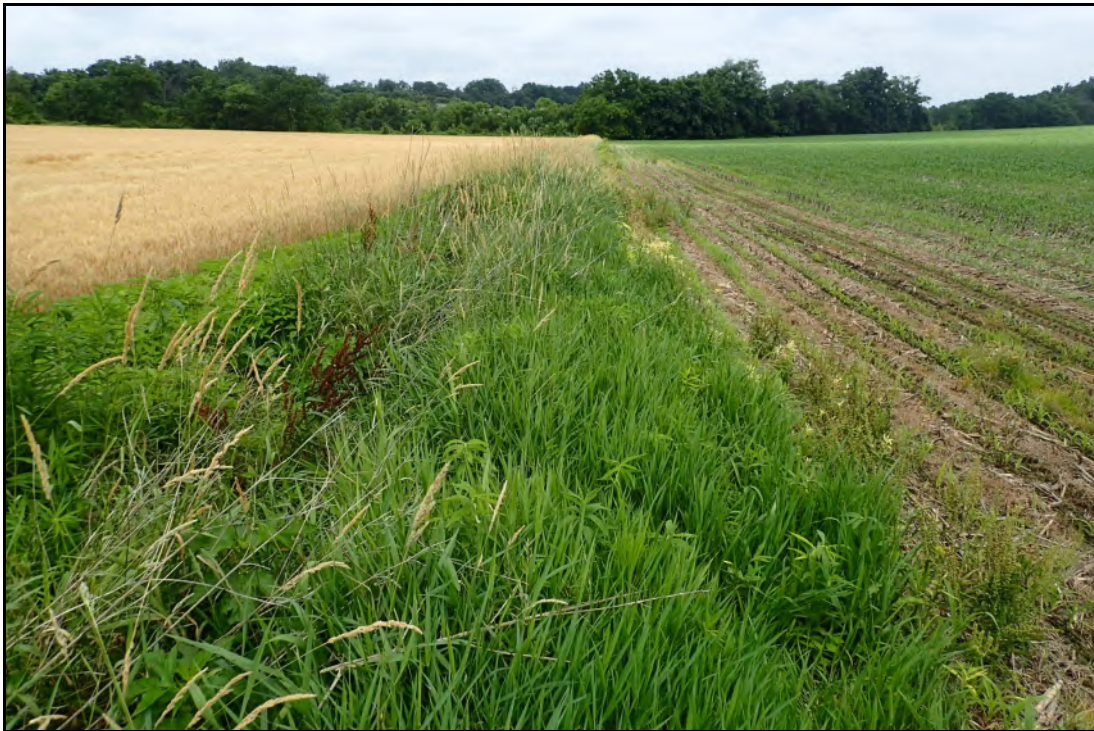
Appendix C4. A second linear, ag-ditch extends northeast to southwest with an eventual intersection with the pond outflow ditch (view faces northeast).
