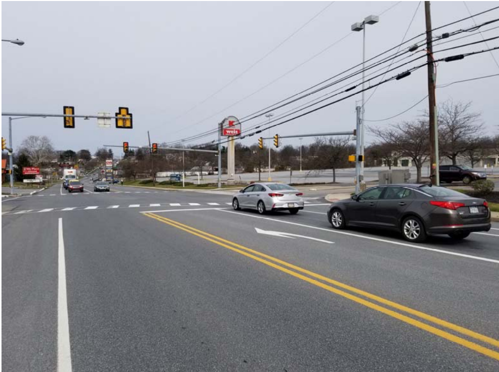
SR 0230 looking west (50') at Hess Driveway/Market Square Driveway
