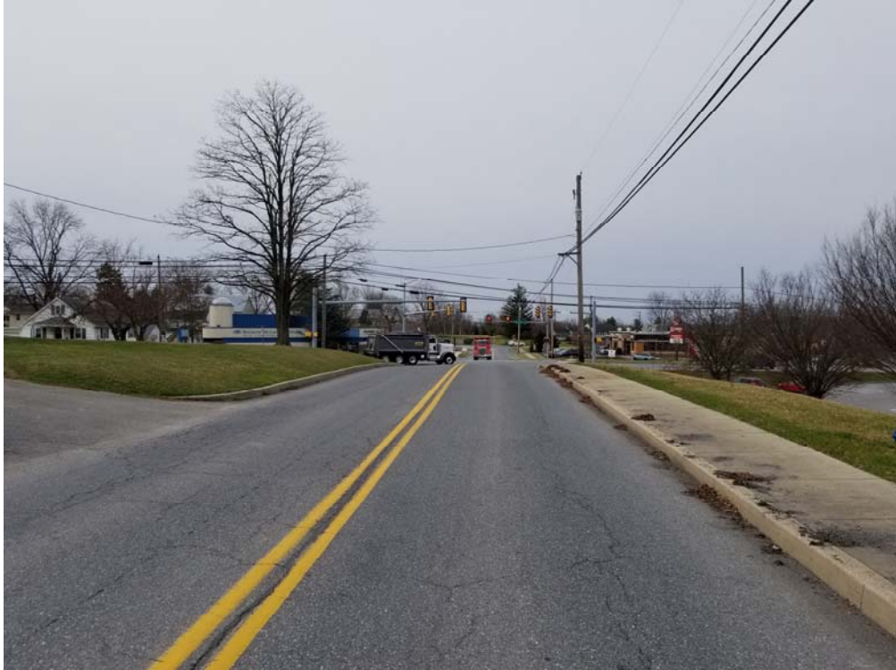
Sheaffer Road looking south (200') at SR 0230
