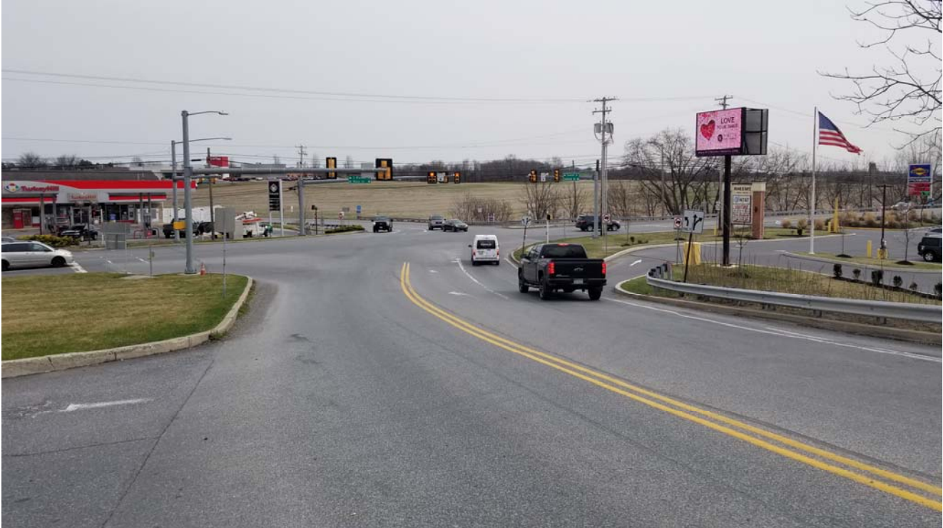
Colebrook Road looking north (200') at SR 0230
