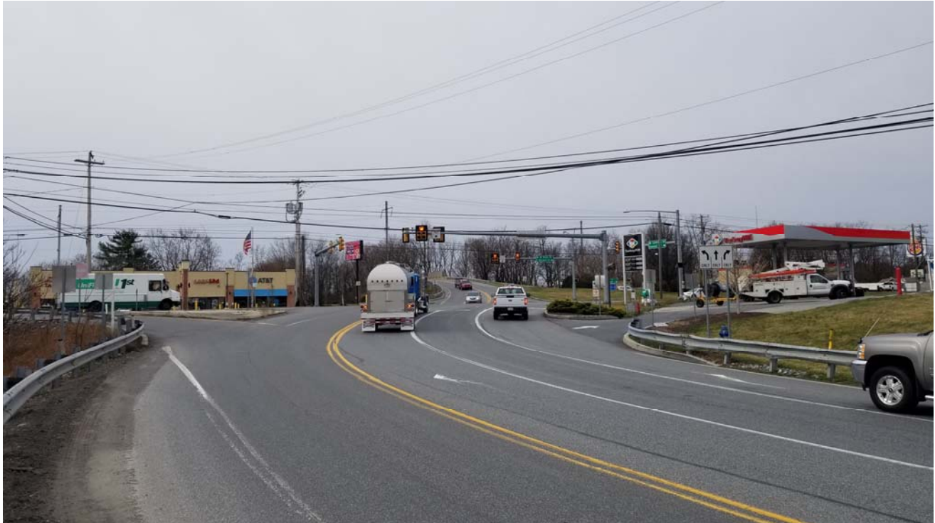
Cloverleaf Road looking south (200') at SR 0230
