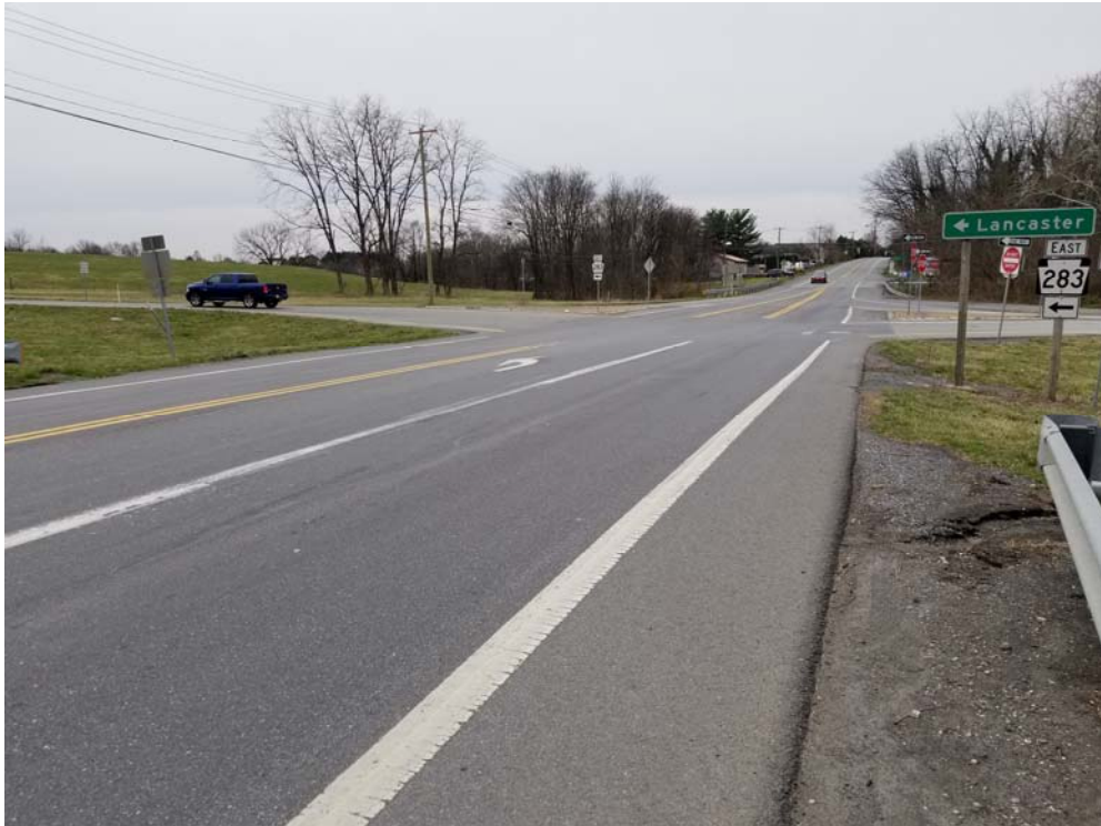
Cloverleaf Road looking south (50') at PA 283 EB Ramps
