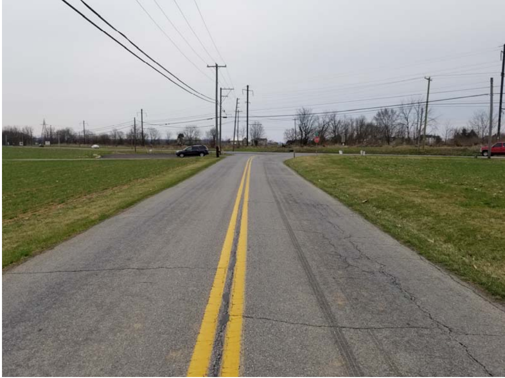
Ridge Run Road looking south (200') at SR 0230
