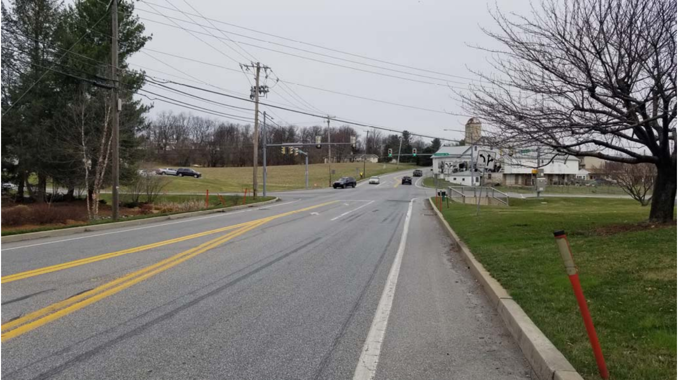
Cloverleaf Road looking north (200') at Schwanger Road
