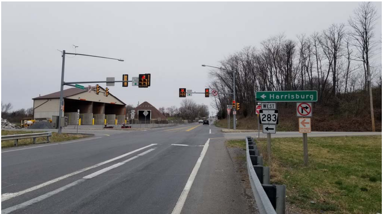
Cloverleaf Road looking north (50') at PA 283 WB Ramps
