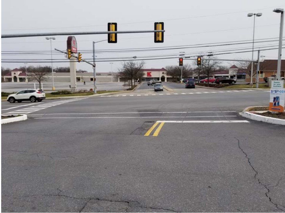
Hess Driveway looking north at SR 0230
