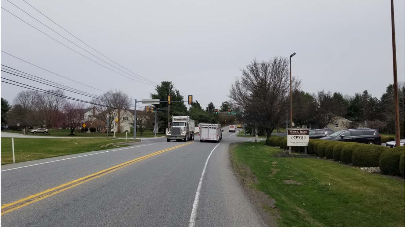
Cloverleaf Road looking north (200') at Andrew Avenue/Norlanco Drive
