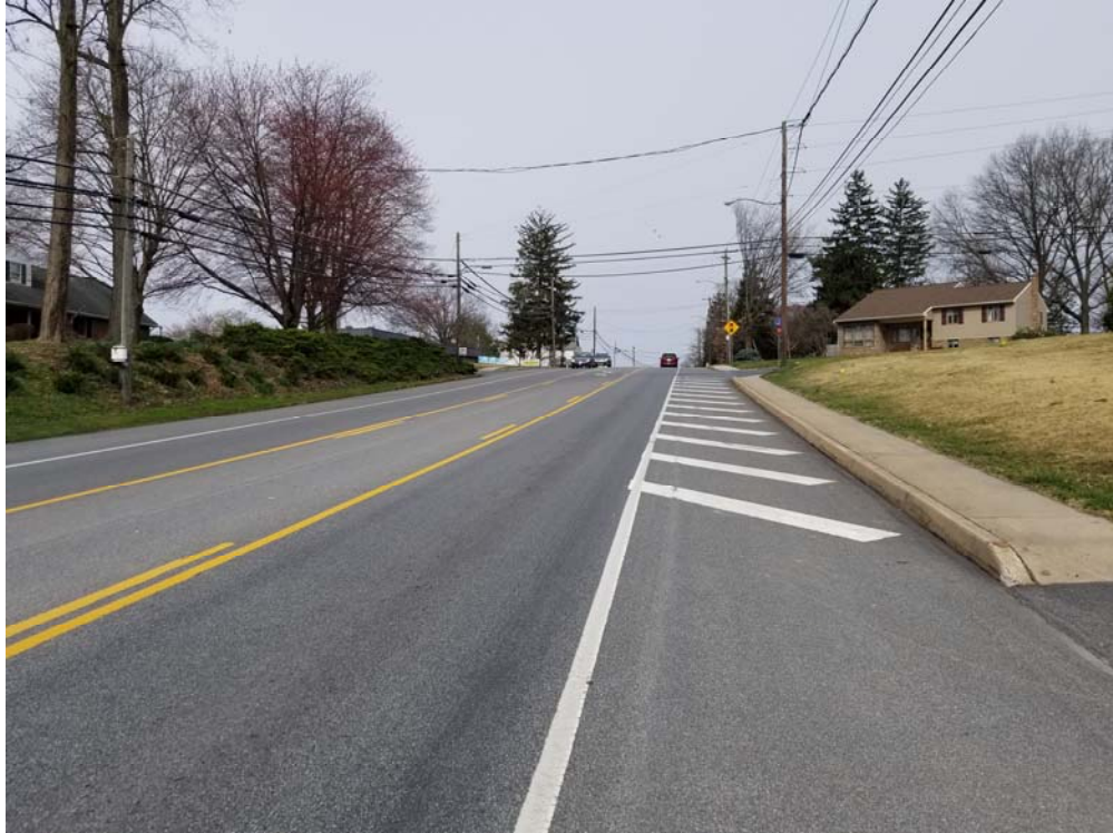
SR 0230 looking west (200') at Groff Avenue
