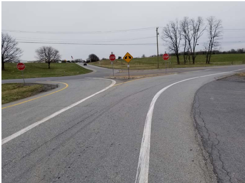
PA 283 EB Ramps looking east (50') at Cloverleaf Road
