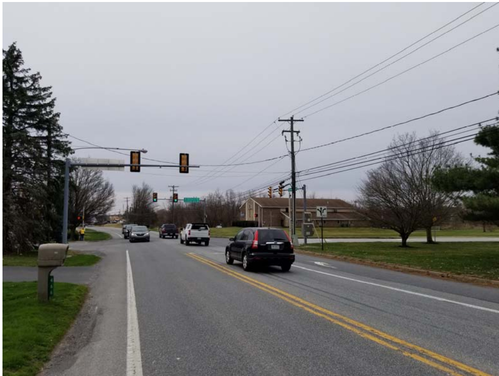
Cloverleaf Road looking south (50') at Andrew Avenue/Norlanco Drive
