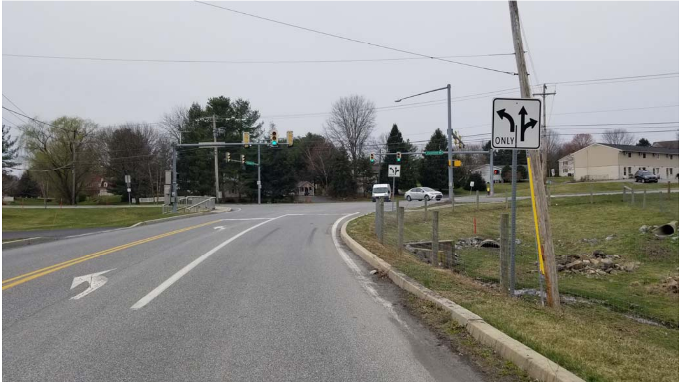
Schwanger Road looking west (200') at Cloverleaf Road
