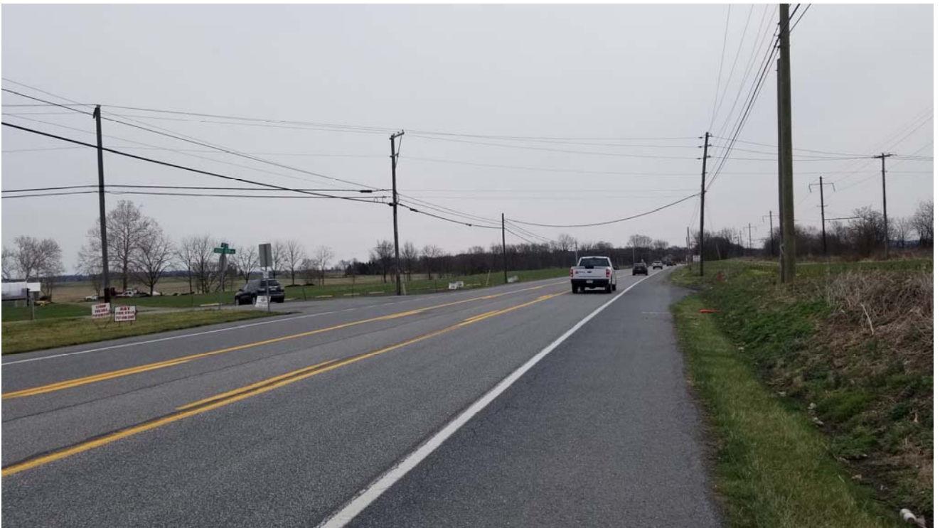
SR 0230 looking east (50') at Ridge Run Road
