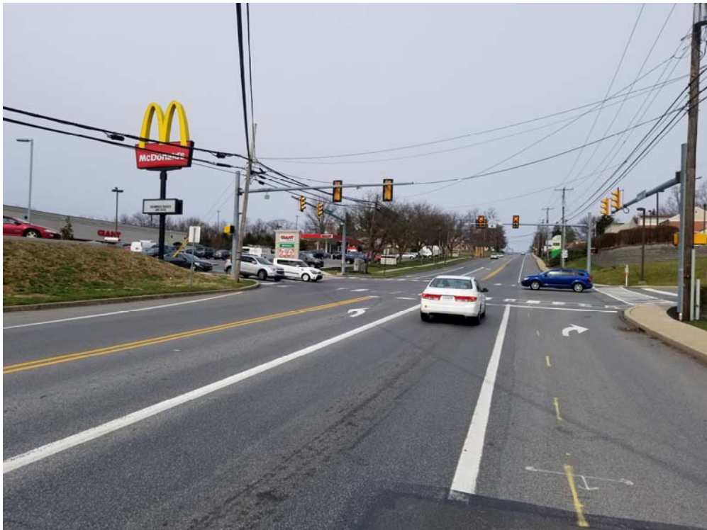
SR 0230 looking west (50') at Carey Lane/Giant Plaza Driveway
