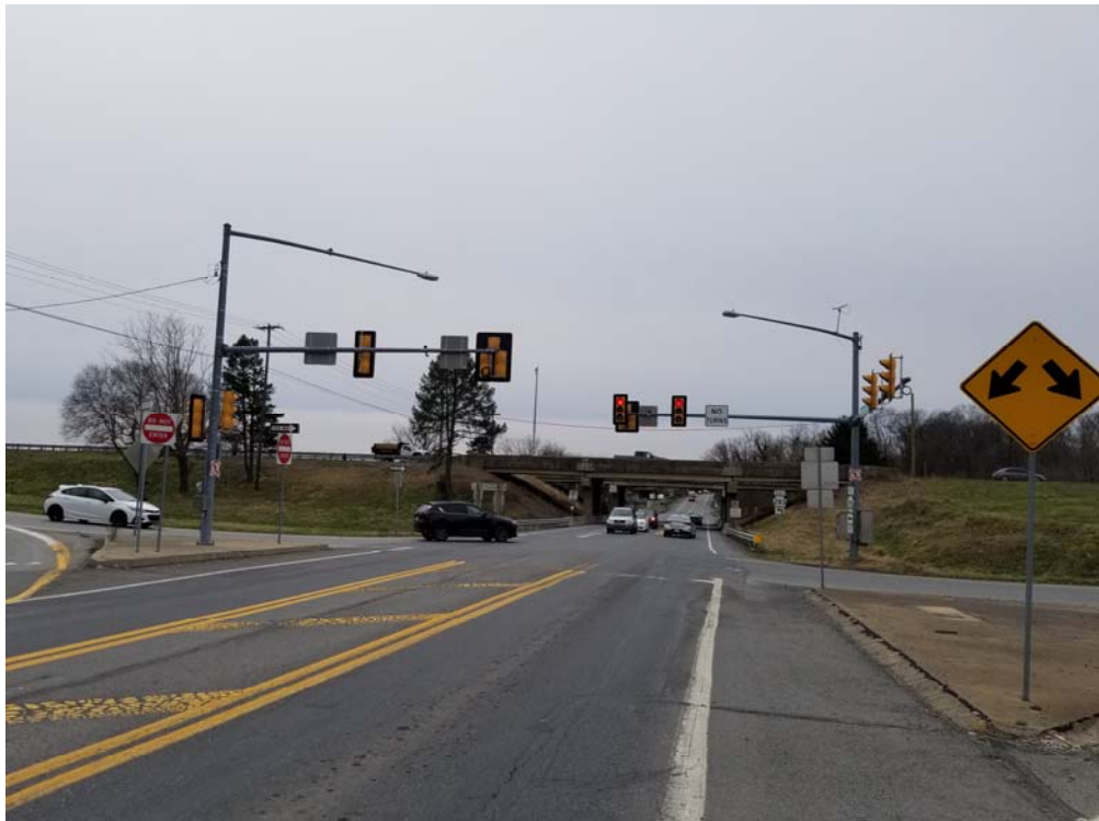
Cloverleaf Road looking south (50') at PA 283 WB Ramps
