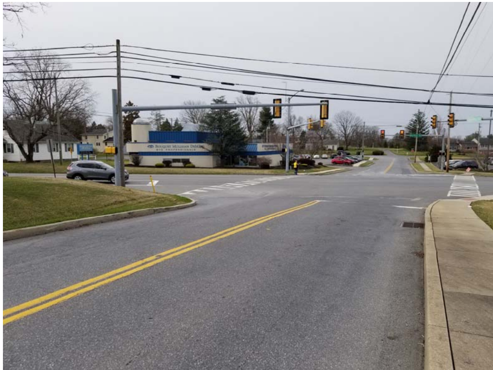
Sheaffer Road looking south (50') at SR 0230
