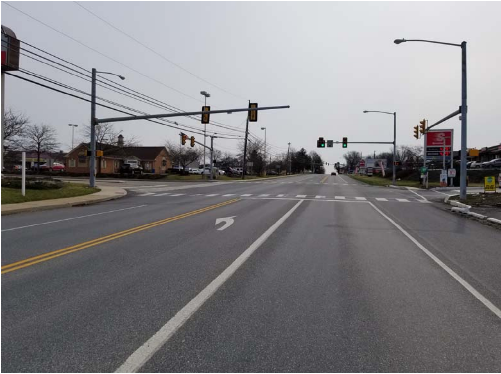
SR 0230 looking east (50') at Hess Driveway/Market Square Driveway
