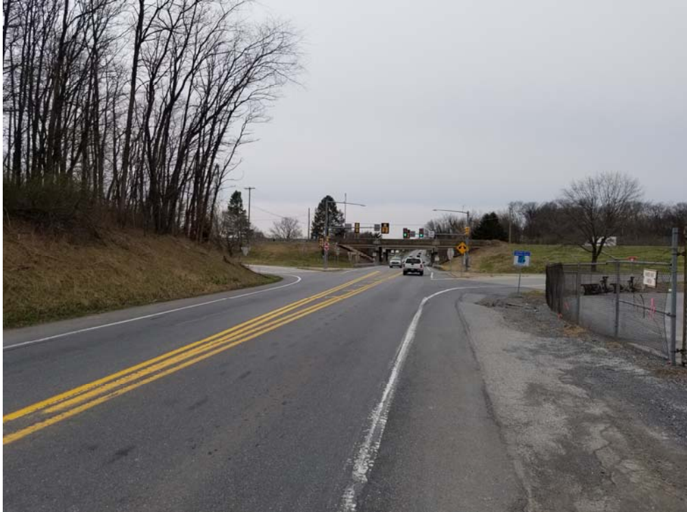
Cloverleaf Road looking south (200') at PA 283 WB Ramps
