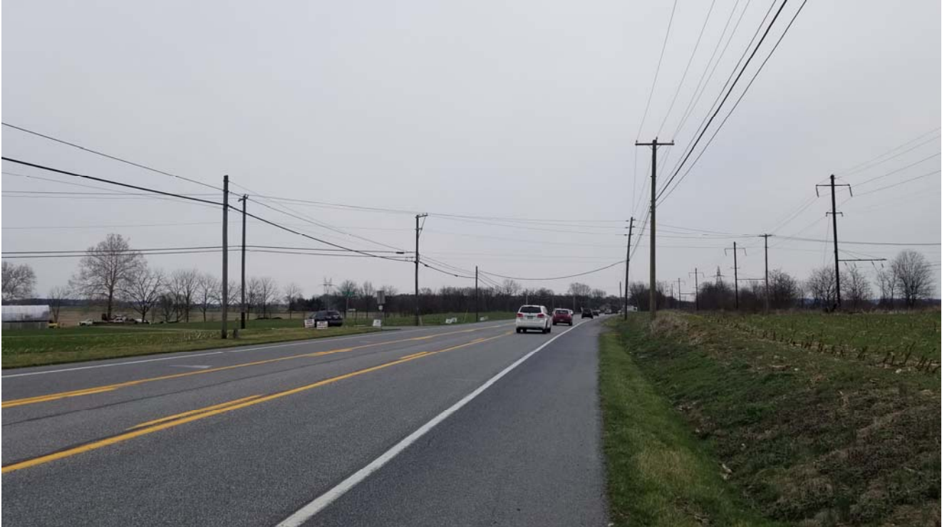
SR 0230 looking east (200') at Ridge Run Road
