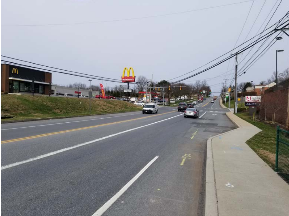
SR 0230 looking west (200') at Carey Lane/Giant Plaza Driveway
