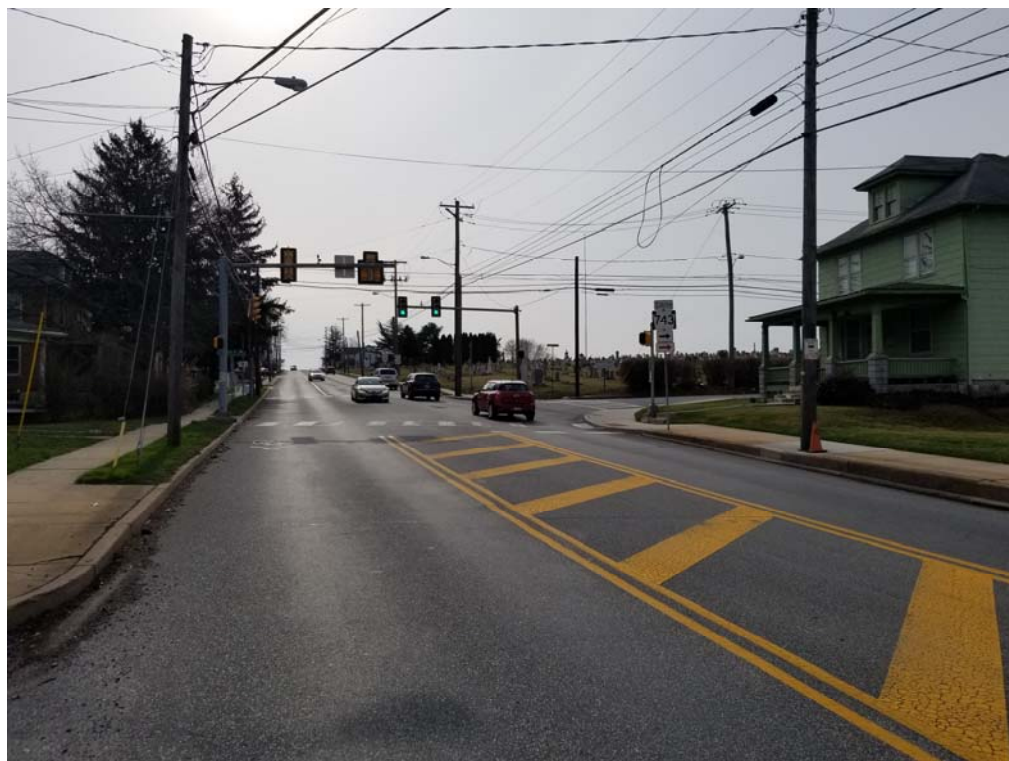
SR 0230 looking east (50') at SR 0743
