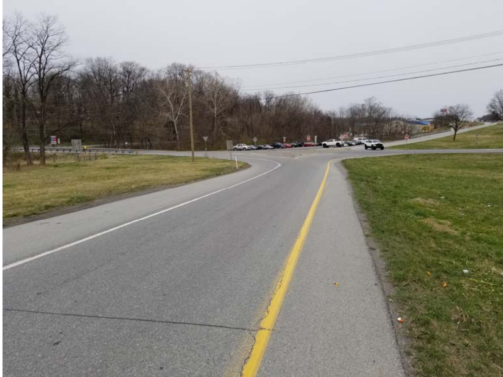
PA 283 EB Ramps looking west (200') at Cloverleaf Road
