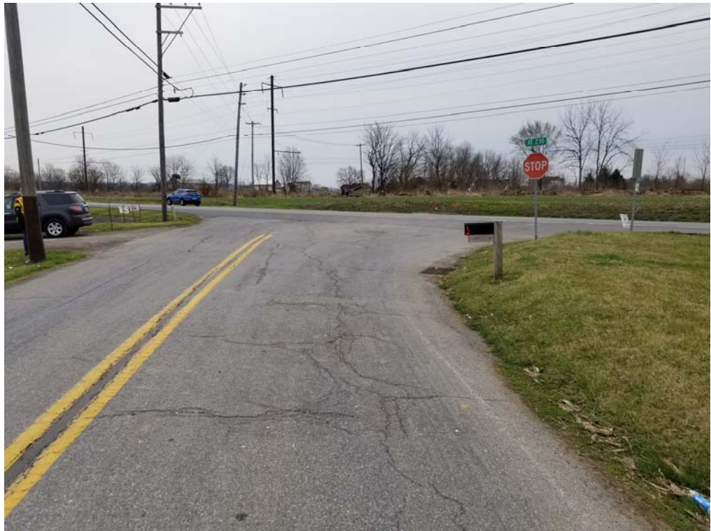
Ridge Run Road looking south (50') at SR 0230
