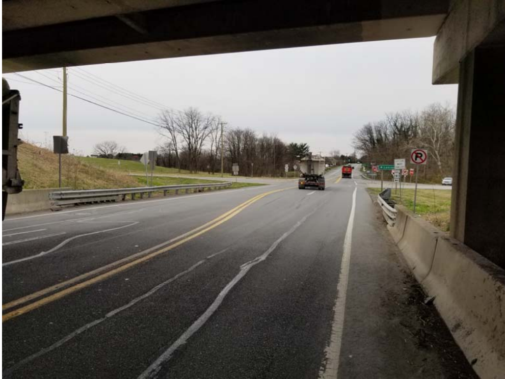
Cloverleaf Road looking south (200') at PA 283 EB Ramps
