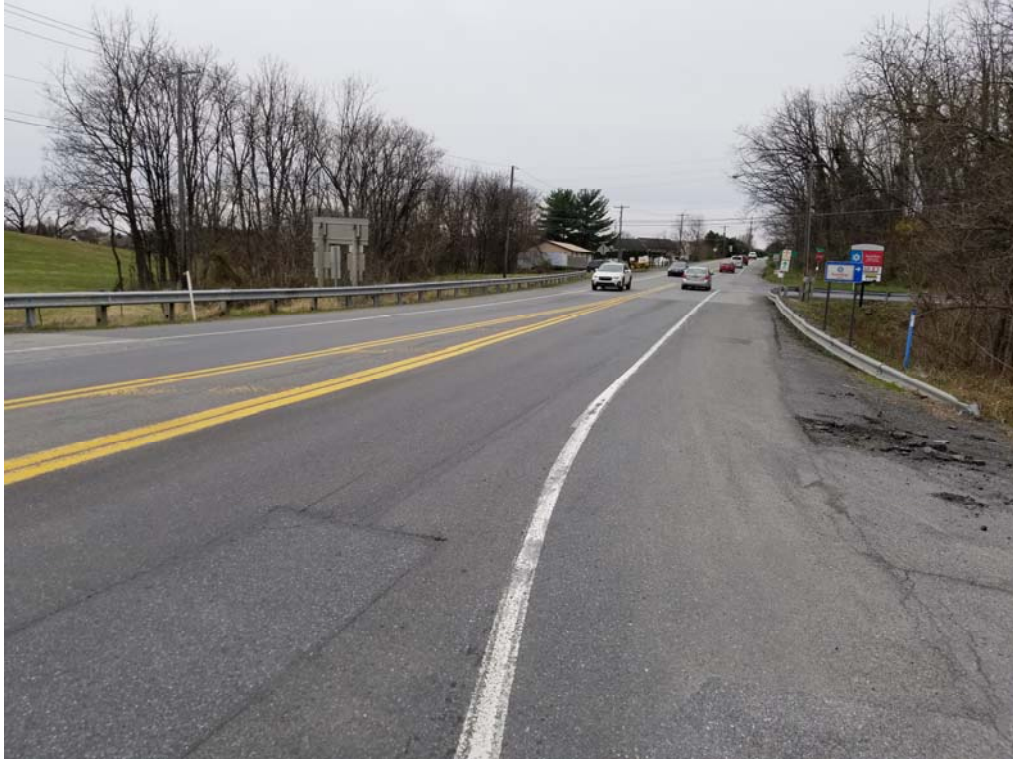
Cloverleaf Road looking south (200') at Merts Drive
