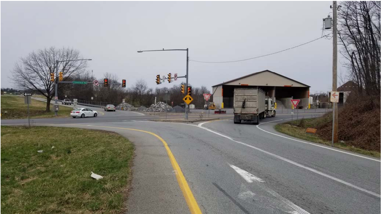
PA 283 WB Ramps looking west (50') at Cloverleaf Road
