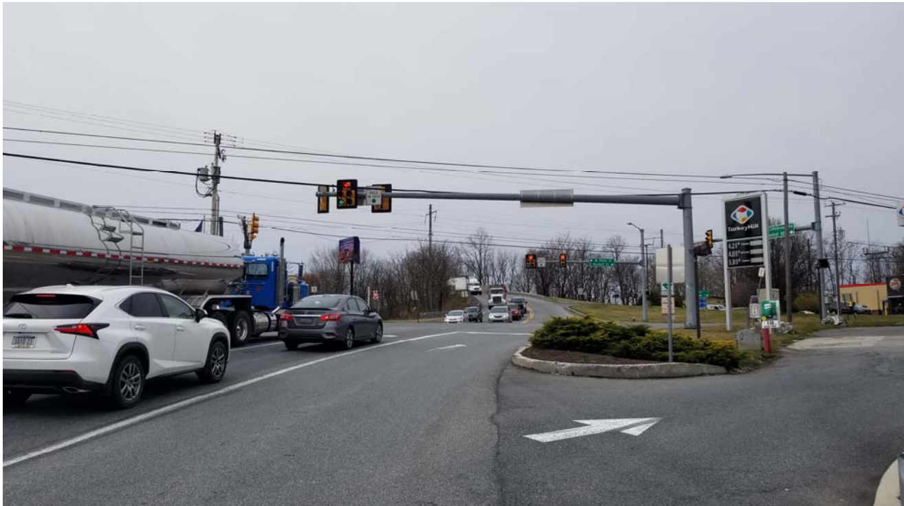
Cloverleaf Road looking south (50') at SR 0230
