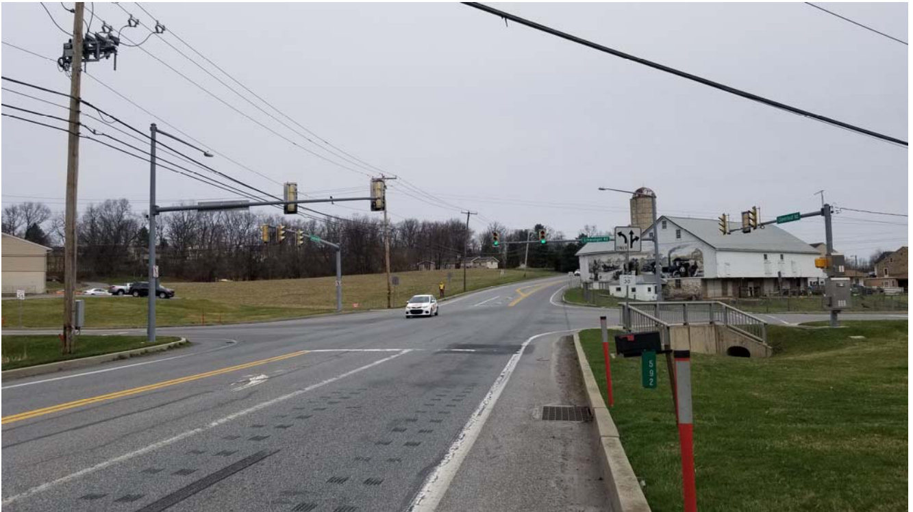
Cloverleaf Road looking north (50') at Schwanger Road
