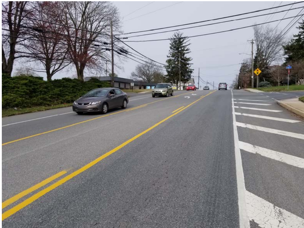
SR 0230 looking west (50') at Groff Avenue
