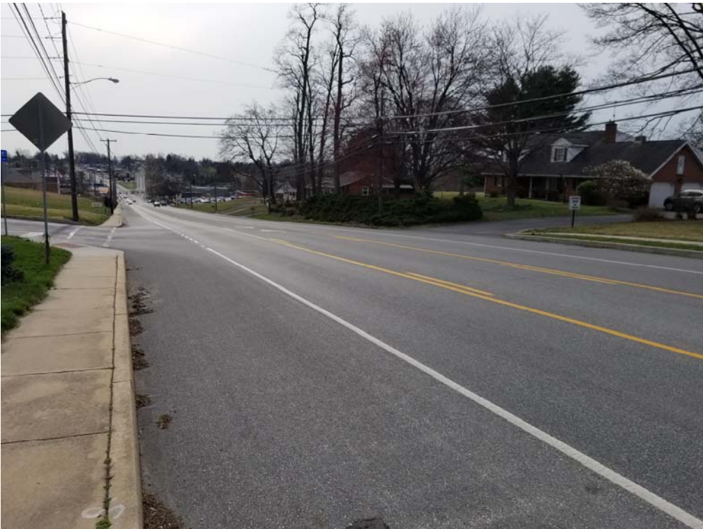
SR 0230 looking east (50') at Groff Avenue
