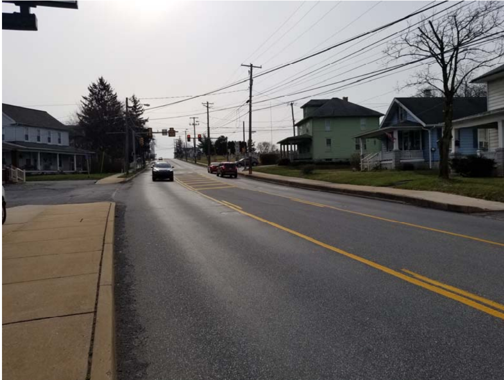
SR 0230 looking east (200') at SR 0743
