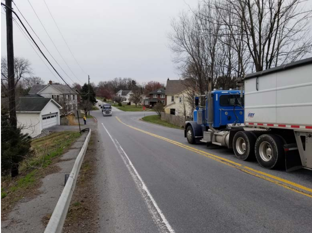
Colebrook Road looking south (200') at Harrisburg Avenue
