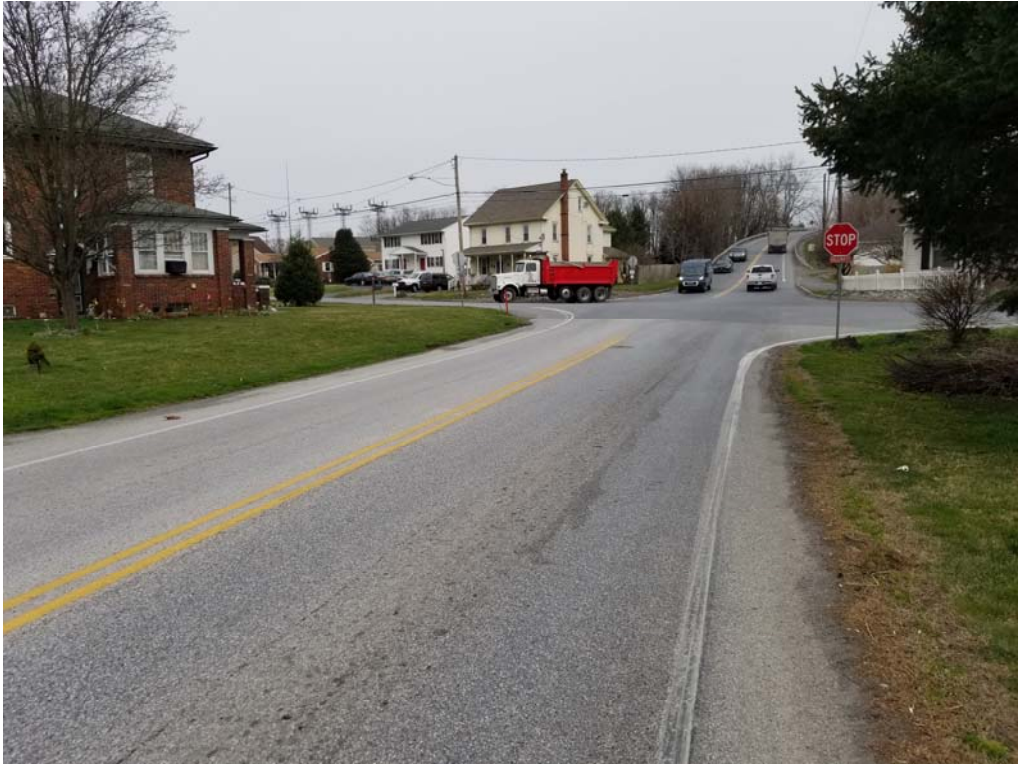
Colebrook Road looking north (50') at Harrisburg Avenue
