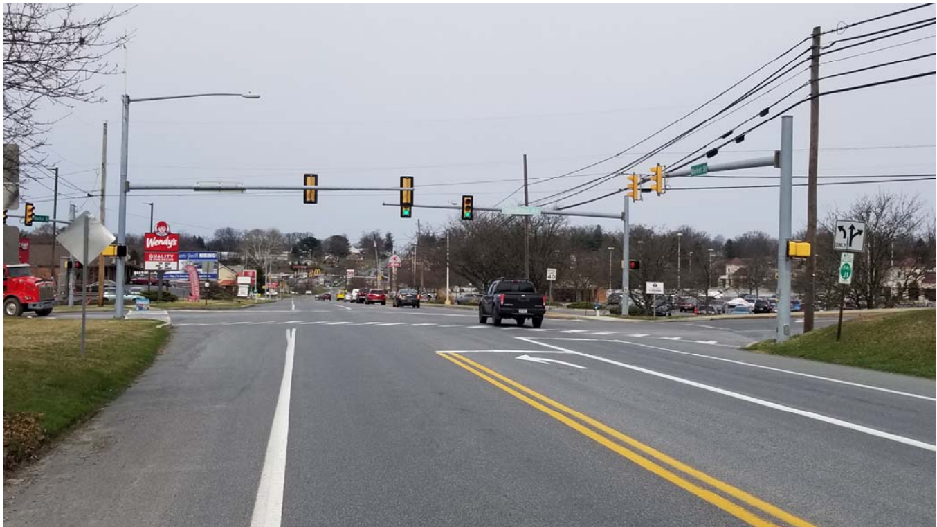
SR 0230 looking west (50') at Sheaffer Road
