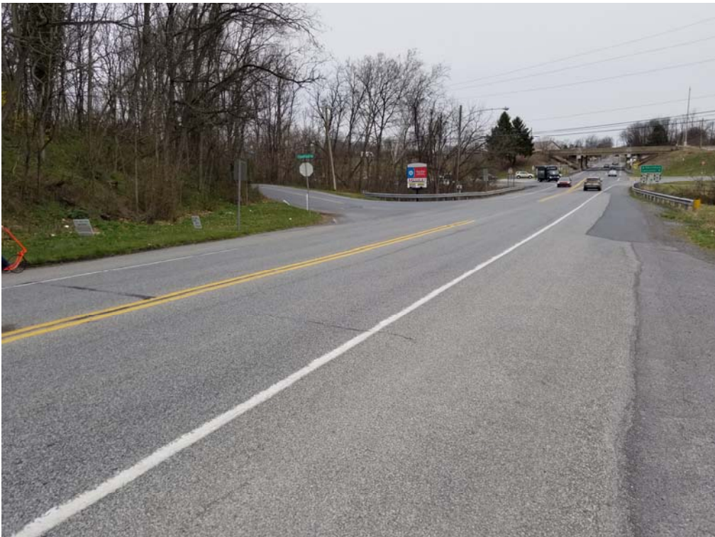
Cloverleaf Road looking north (50') at Merts Drive
