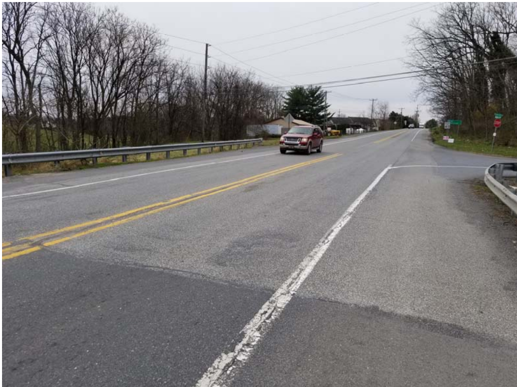
Cloverleaf Road looking south (50') at Merts Drive
