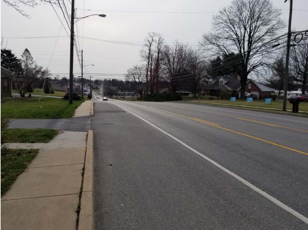
SR 0230 looking east (200') at Groff Avenue
