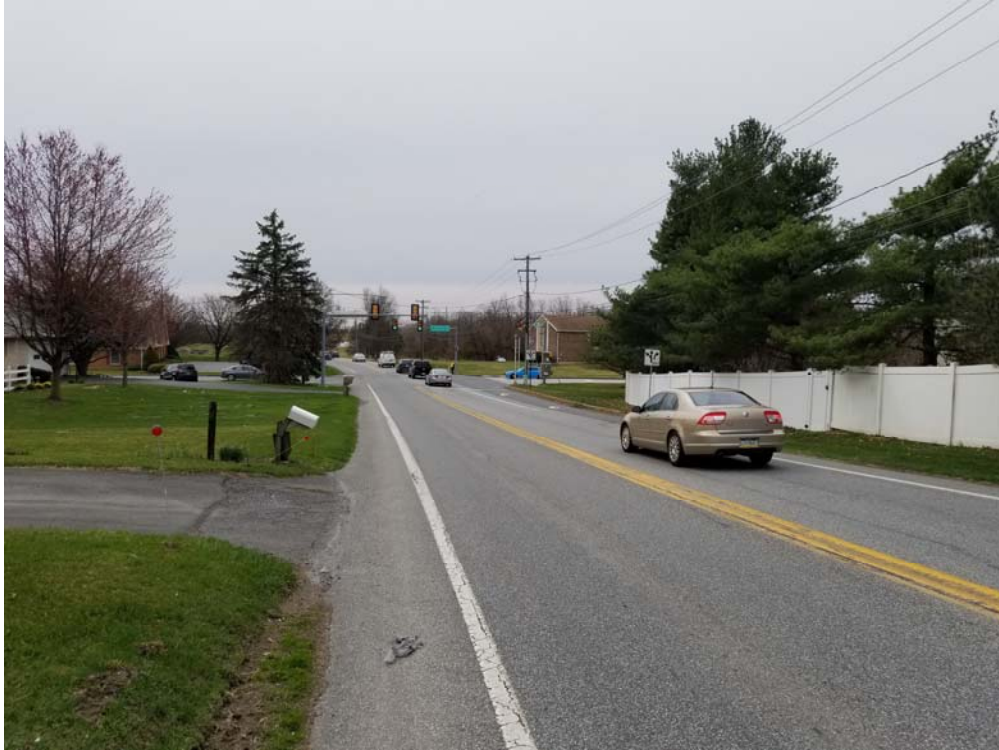
Cloverleaf Road looking south (200') at Andrew Avenue/Norlanco Drive
