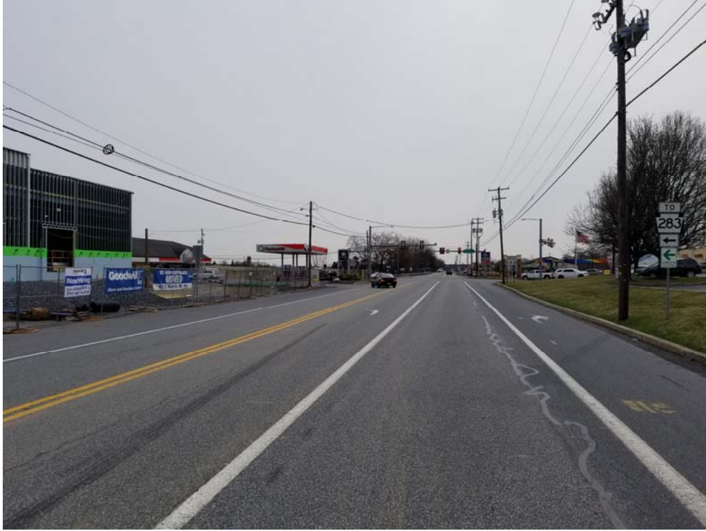
SR 0230 looking east (200') at Cloverleaf Road
