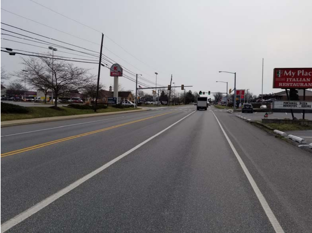
SR 0230 looking east (200') at Hess Driveway/Market Square Driveway
