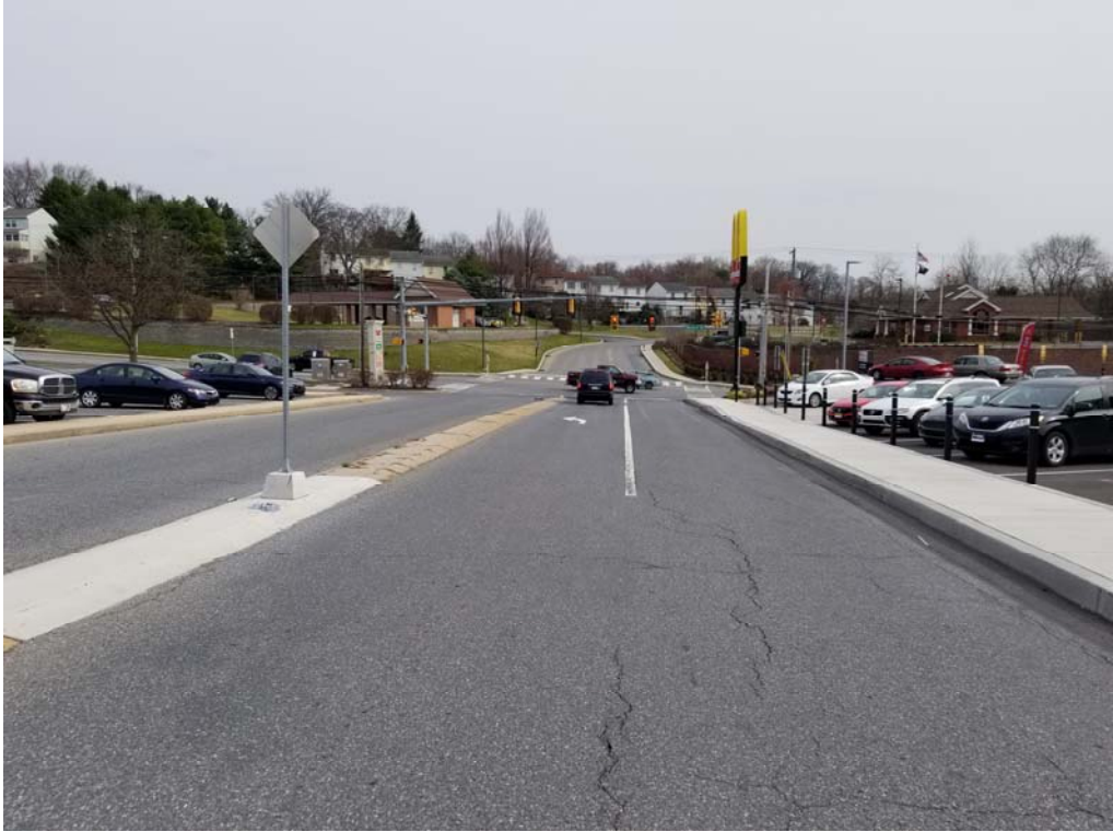
Giant Plaza Driveway looking north (200') at SR 0230
