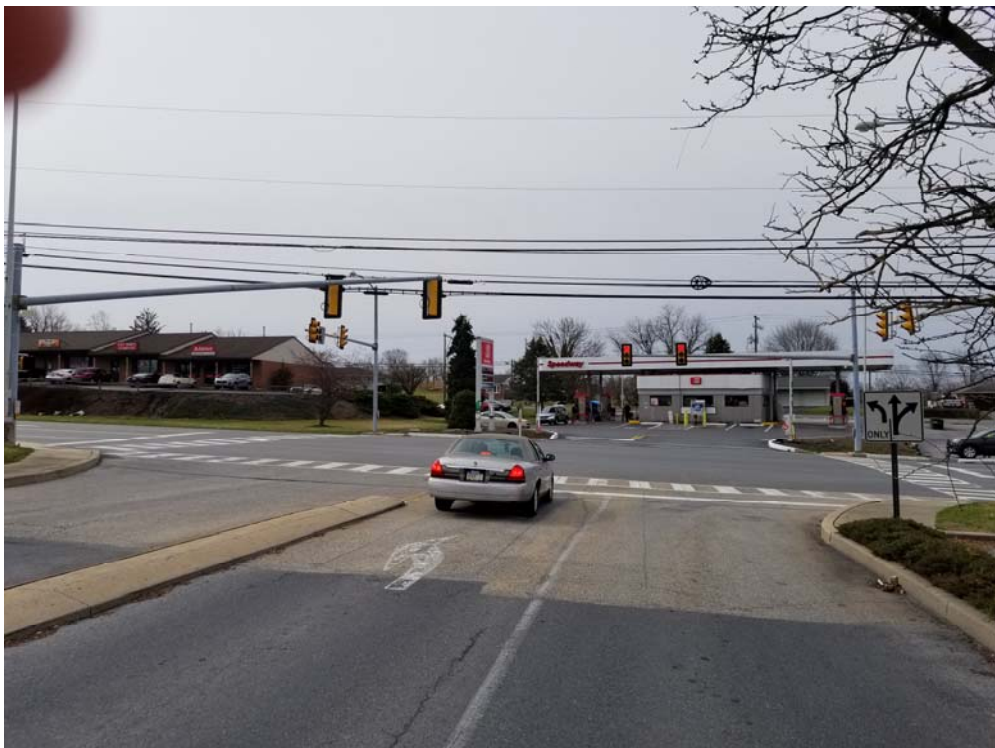
Market Square Driveway looking south (50') at SR 0230
