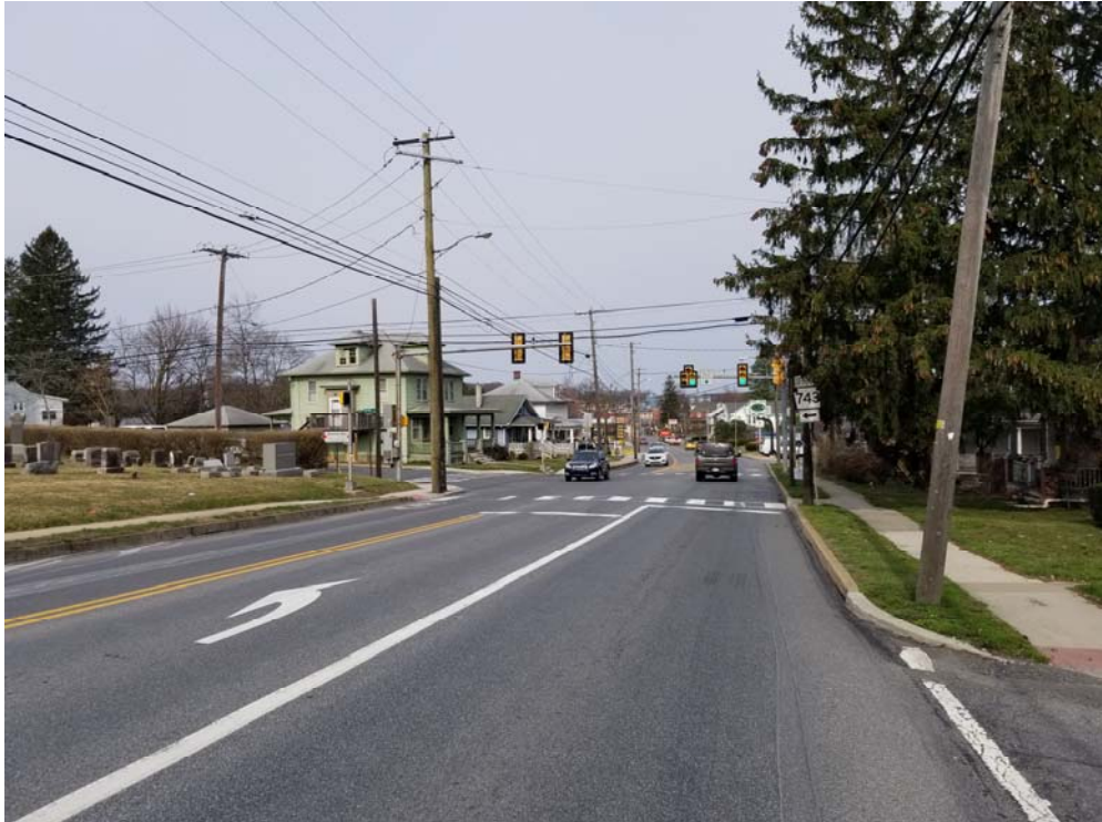
SR 0230 looking west (50') at SR 0743
