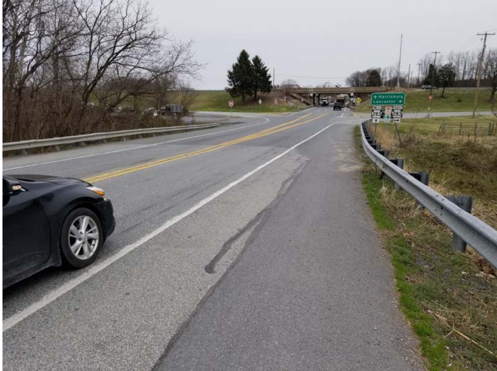
Cloverleaf Road looking north (200') at PA 283 EB Ramps
