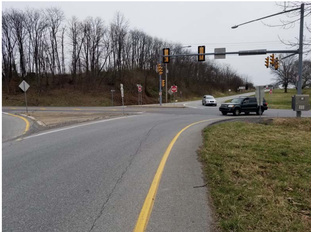
PA 283 WB Ramps looking east (50') at Cloverleaf Road
