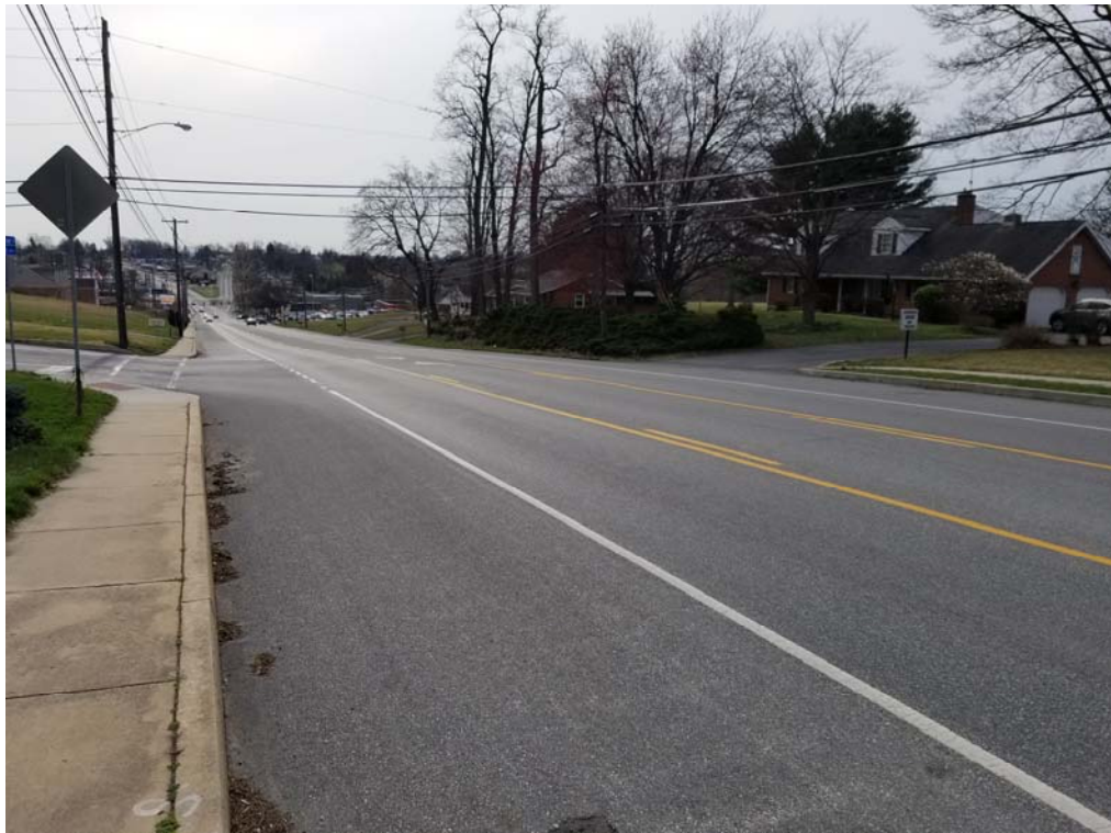
SR 0230 looking east (50') at Groff Avenue
