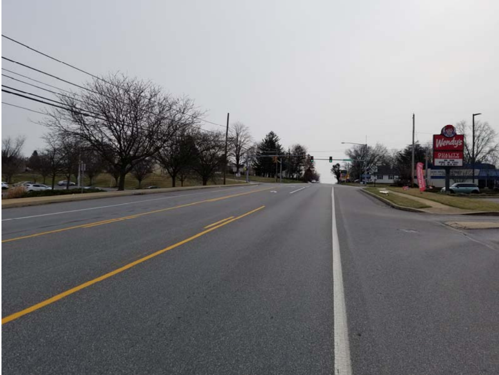
SR 0230 looking east (200') at Sheaffer Road
