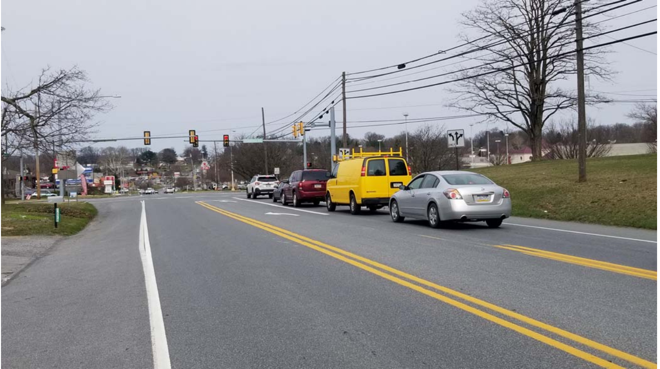
SR 0230 looking west (200') at Sheaffer Road
