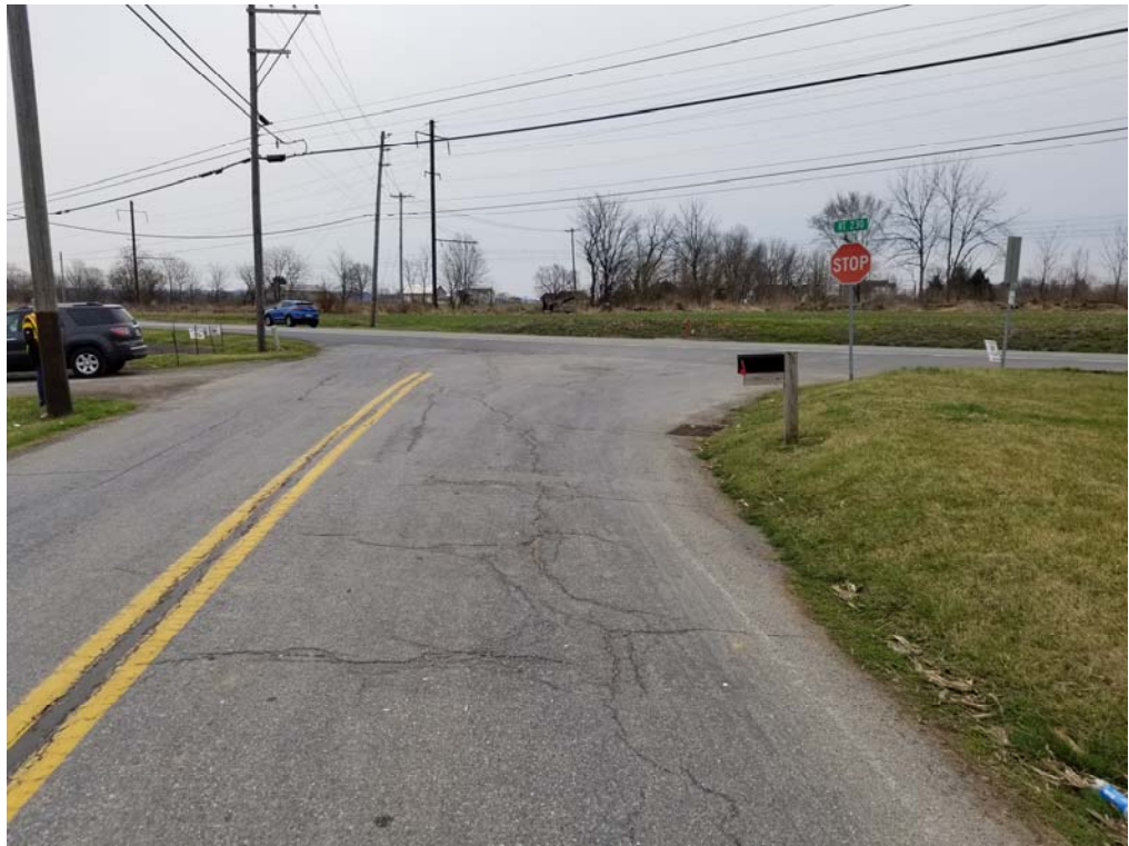
Ridge Run Road looking south (50') at SR 0230
