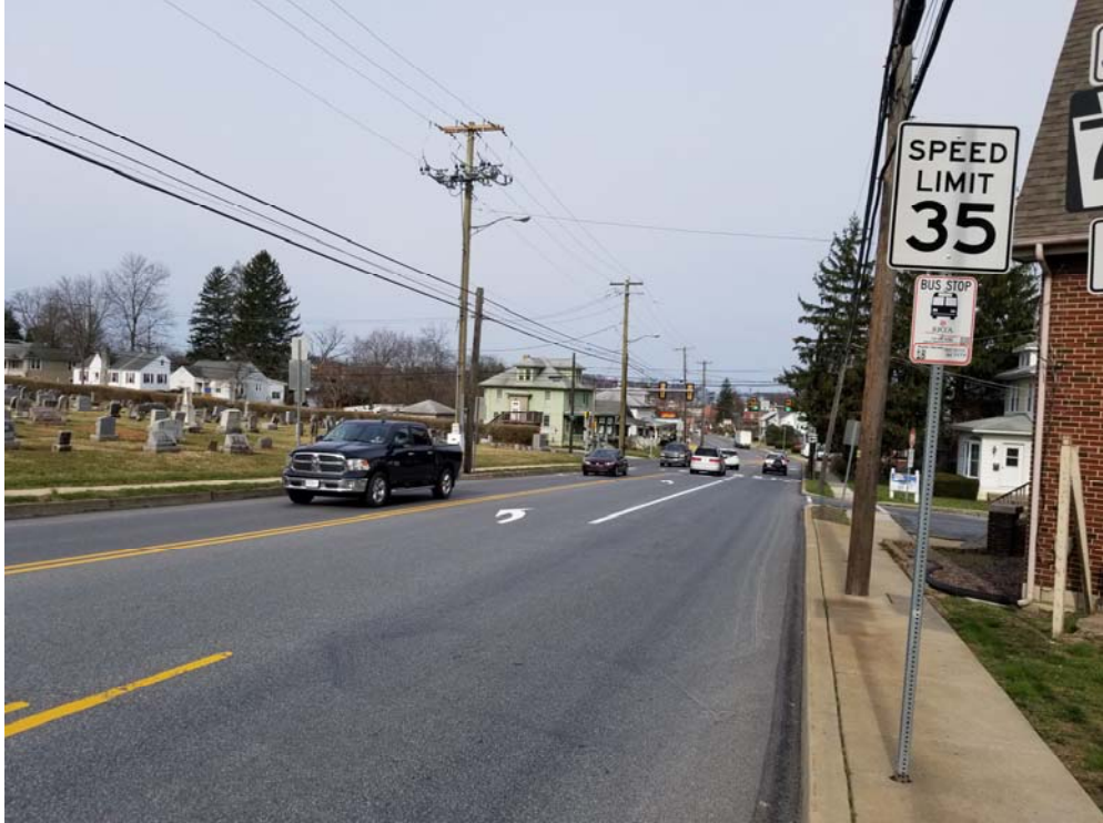
SR 0230 looking west (200') at SR 0743
