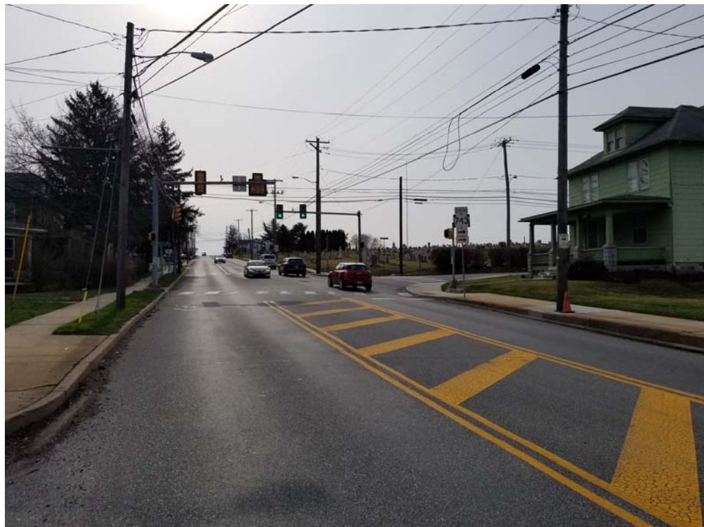
SR 0230 looking east (50') at SR 0743
