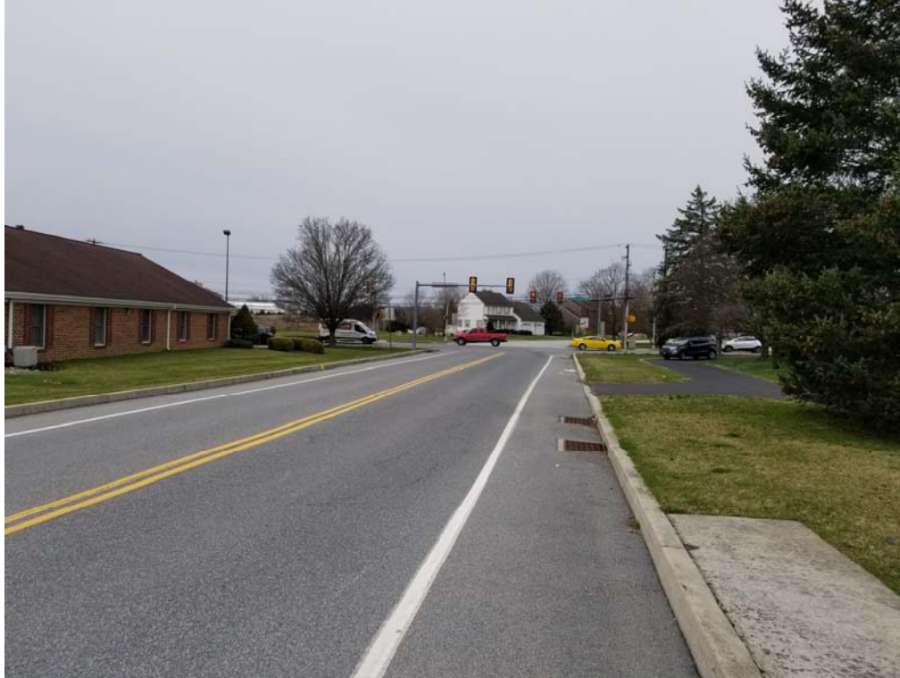
Norlanco Drive looking west (200') at Cloverleaf Road
