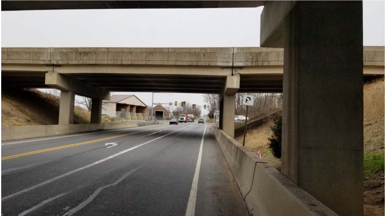
Cloverleaf Road looking north (200') at PA 283 WB Ramps
