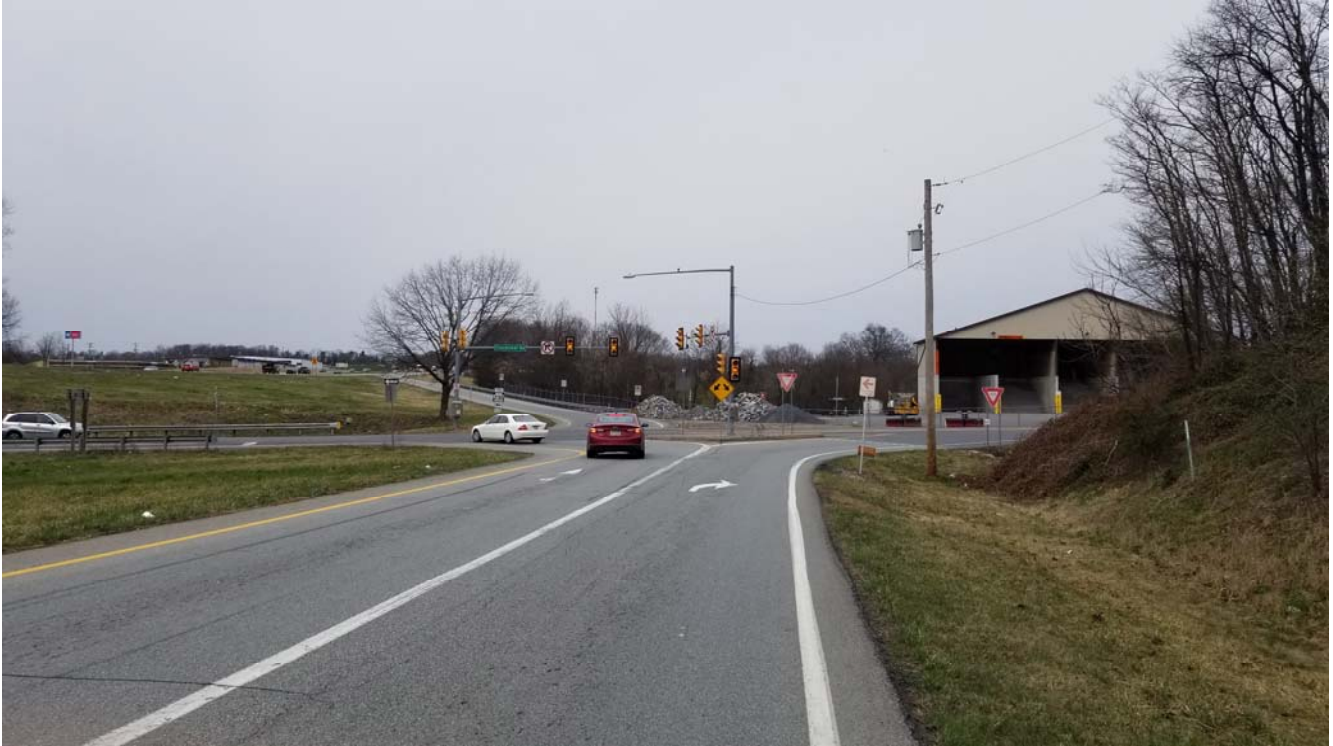
PA 283 WB Ramps looking west (200') at Cloverleaf Road
