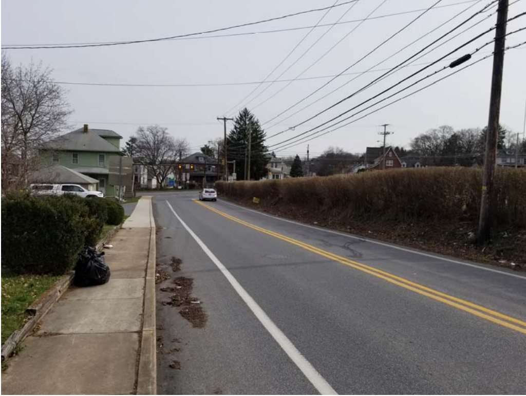
SR 0743 looking north (200') at SR 0230
