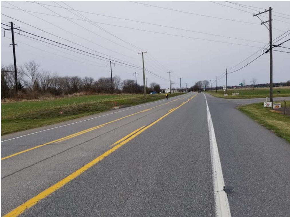
SR 0230 looking west (50') at Ridge Run Road
