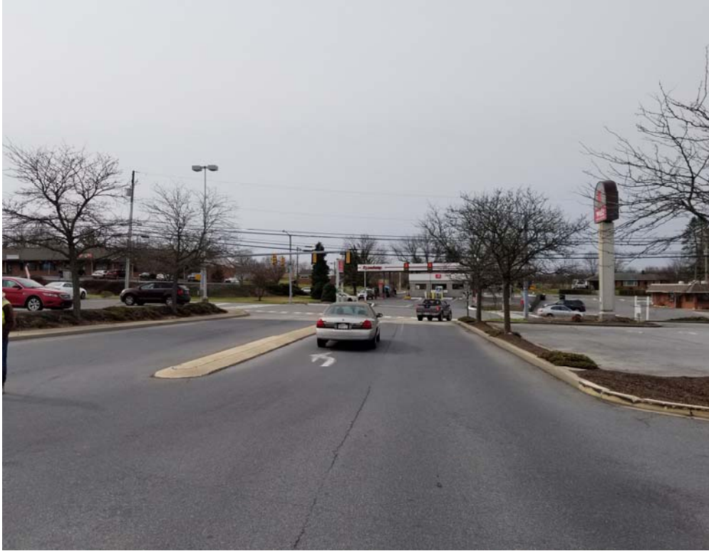
Market Square Driveway looking south (200') at SR 0230
