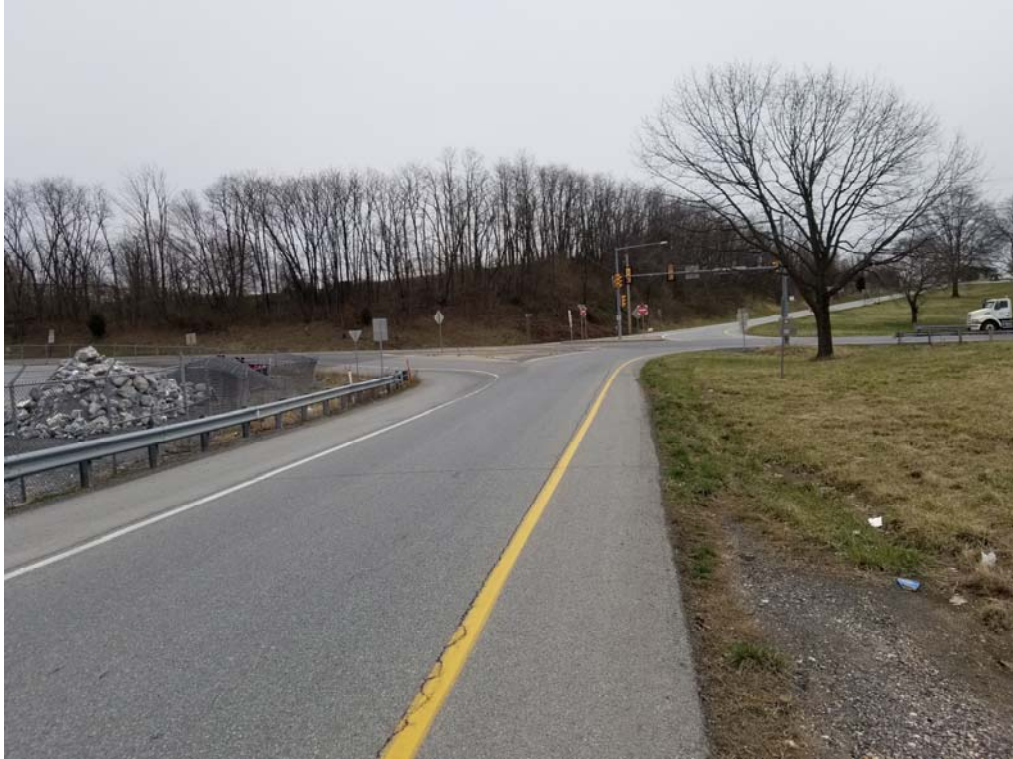
PA 283 WB Ramps looking east (200') at Cloverleaf Road
