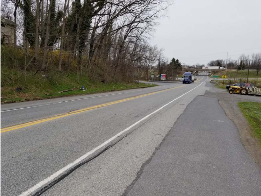
Cloverleaf Road looking north (200') at Merts Drive
