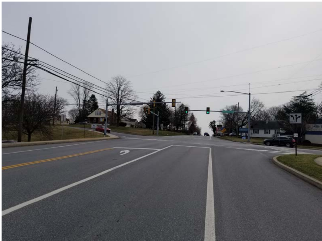
SR 0230 looking east (50') at Sheaffer Road
