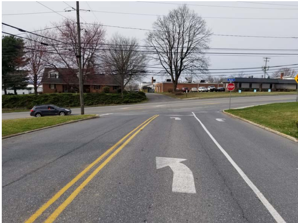
Groff Avenue looking south (50') at SR 0230
