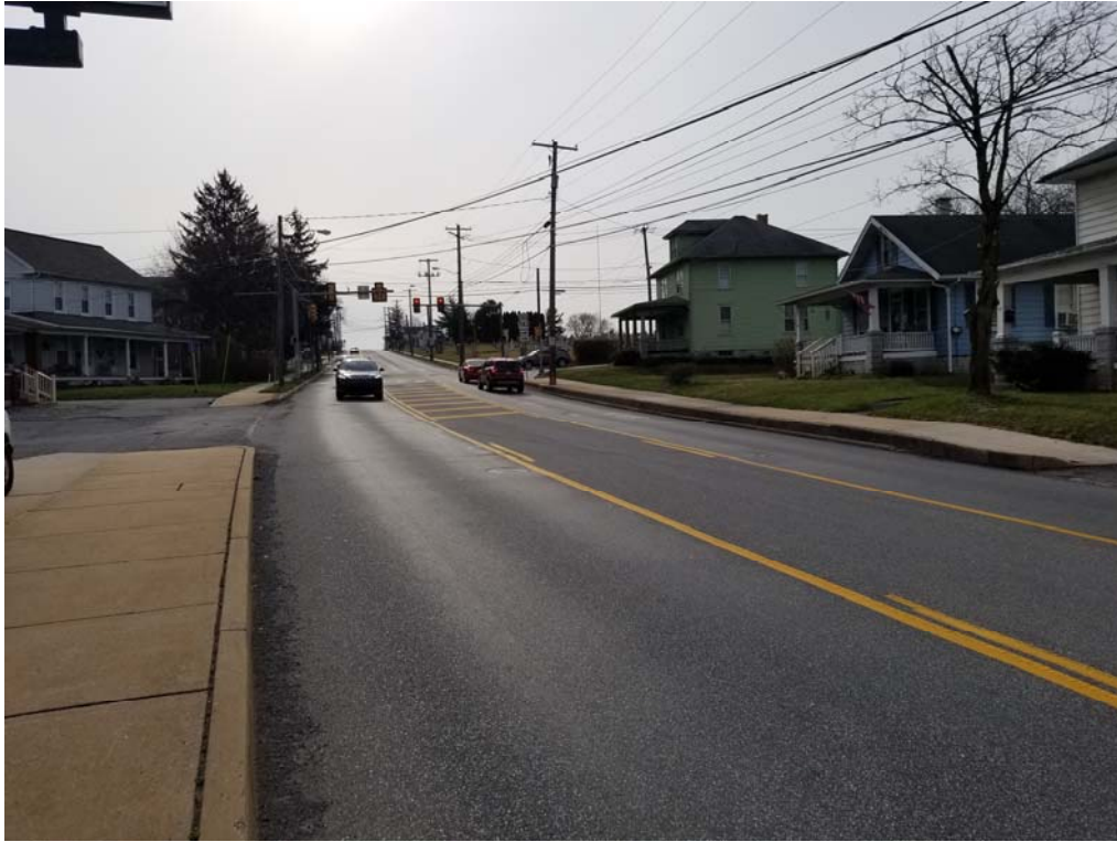
SR 0230 looking east (200') at SR 0743
