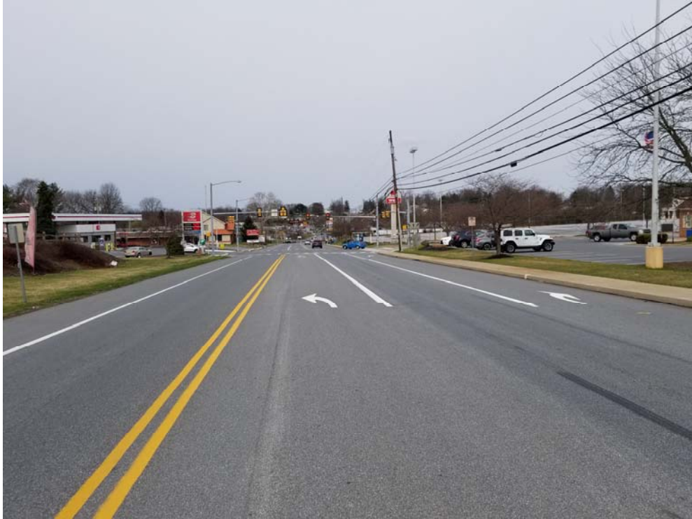
SR 0230 looking west (200') at Hess Driveway/Market Square Driveway
