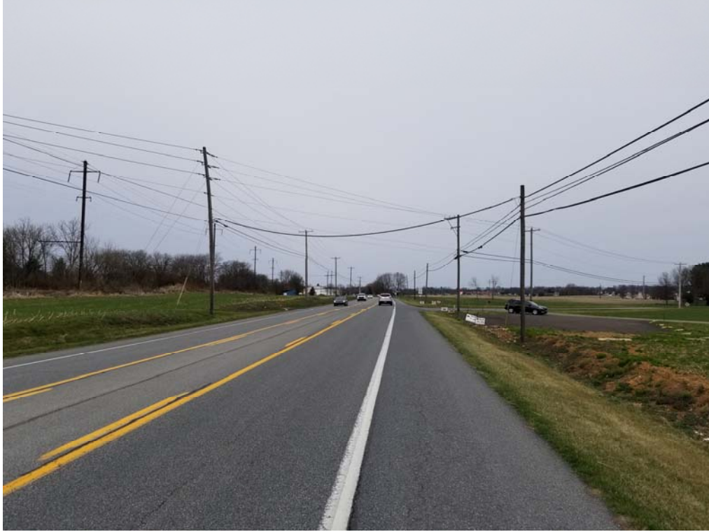
SR 0230 looking west (200') at Ridge Run Road
