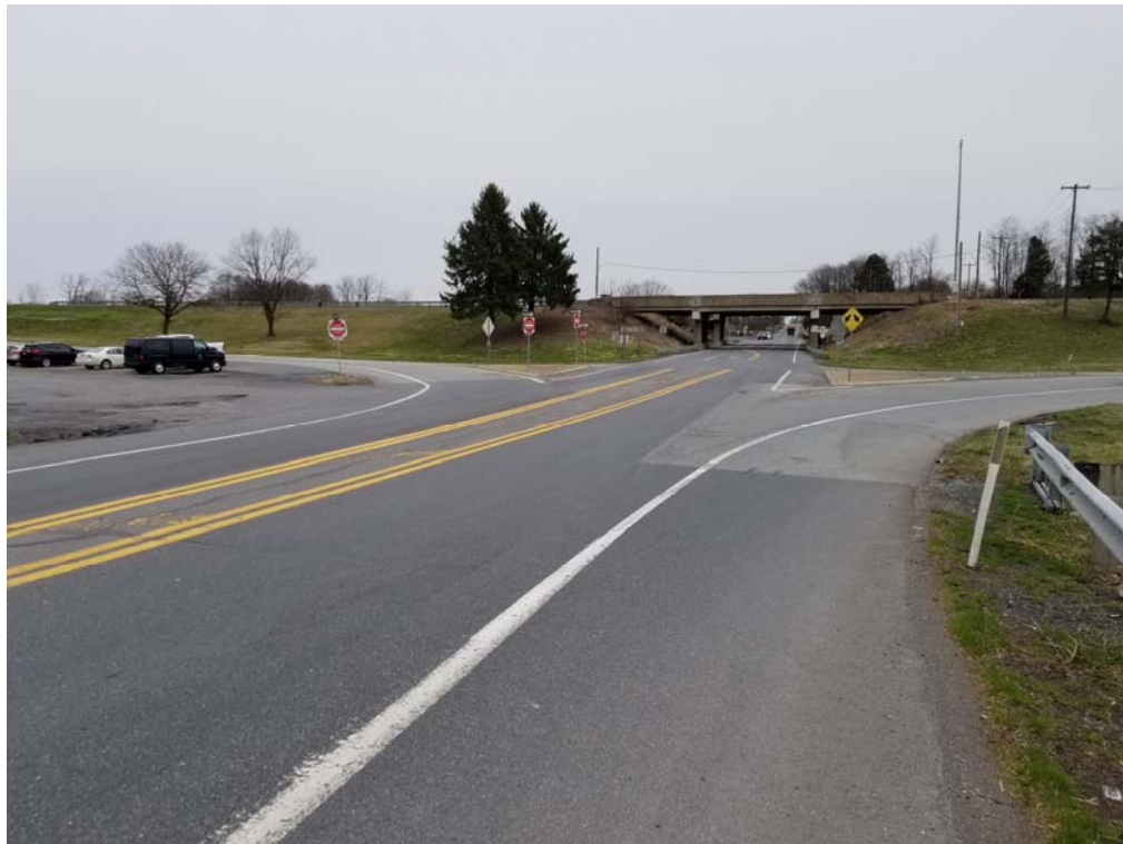
Cloverleaf Road looking north (50') at PA 283 EB Ramps
