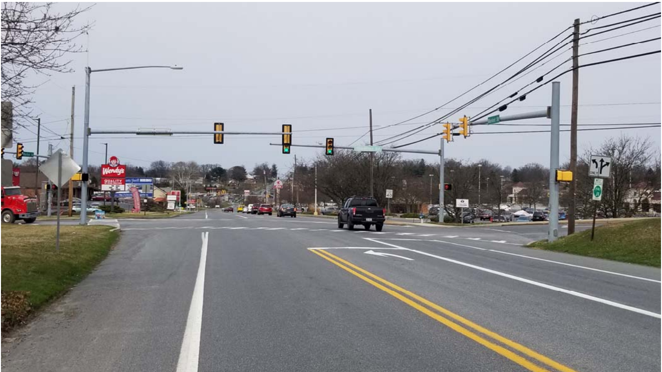
SR 0230 looking west (50') at Sheaffer Road
