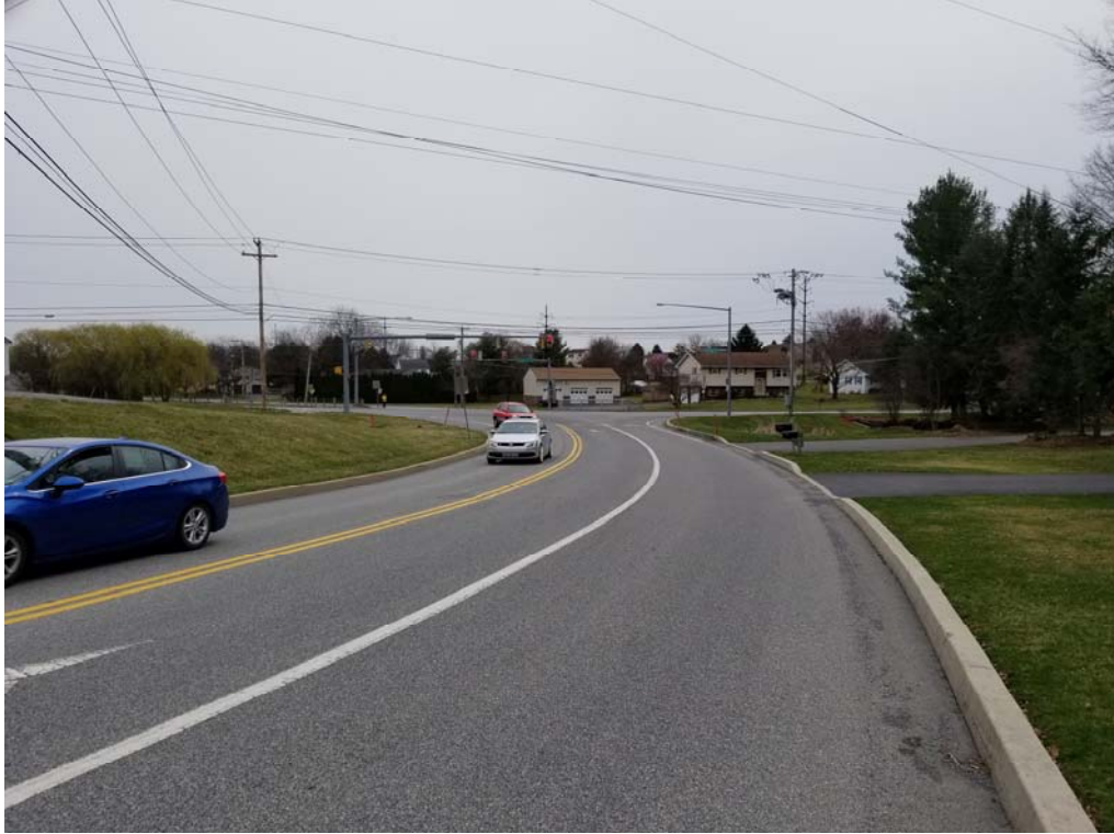
Schwanger Road looking east (200') at Cloverleaf Road
