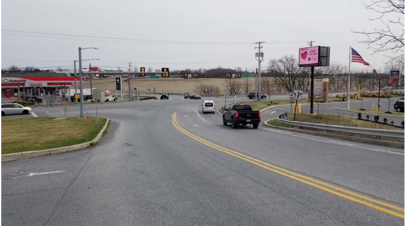
Colebrook Road looking north (200') at SR 0230
