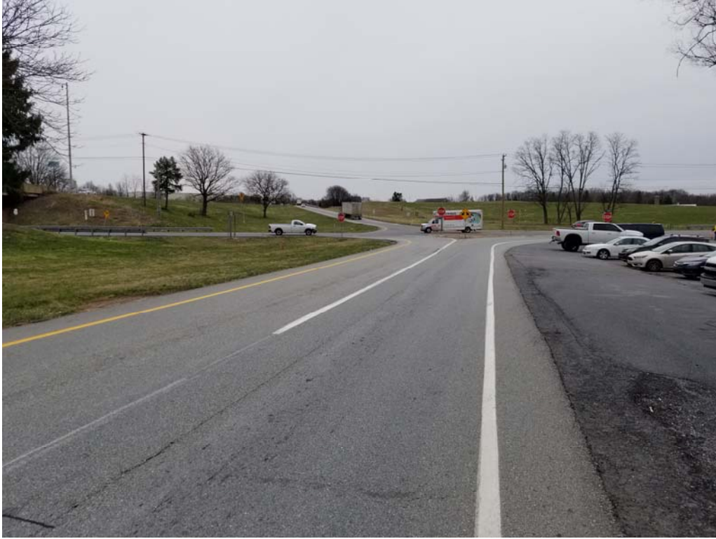
PA 283 EB Ramps looking east (200') at Cloverleaf Road
