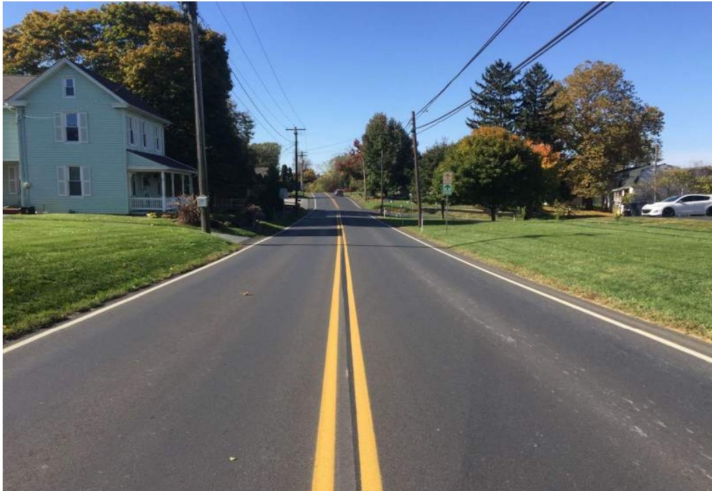
Mt. Joy Road (SR 0772) & Milton Grove Road - WB 200
