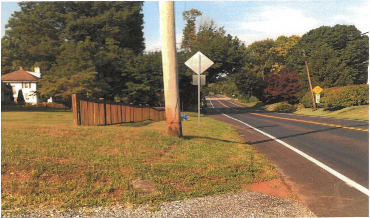
Photo K: Southwestern view along Mt. Joy – Manheim Road (SR 772), which forms the northern boundary of the study area.
