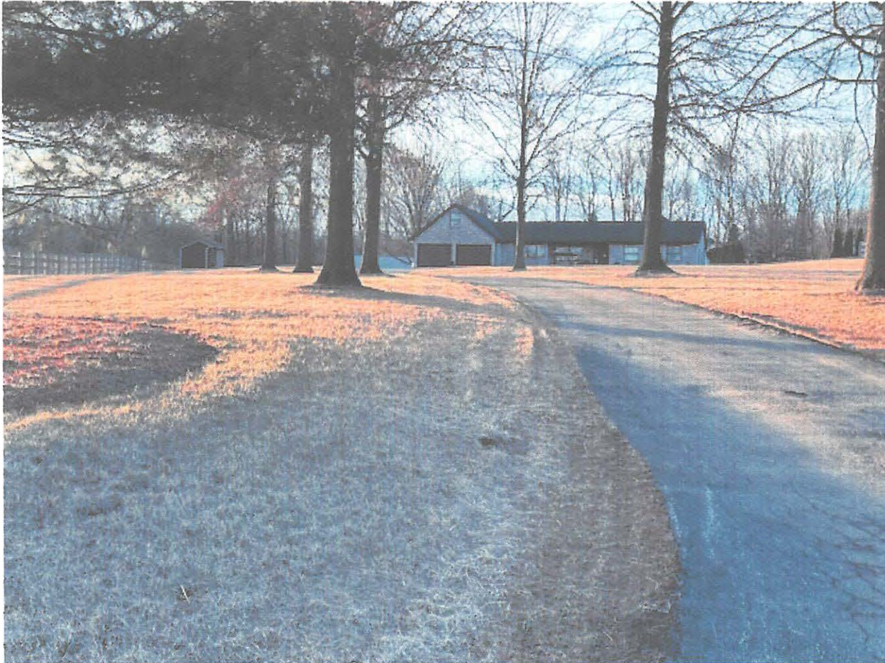
view from street looking back toward storage bins
